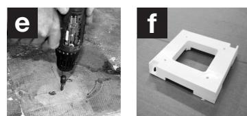
5. Drill platform for plinth anchoring screw [e]. Drive screw to proper depth [f]. Test connection before attaching to post [g]. If using an elevated bracket or aluminum plinth, follow the manufacturers anchoring instructions.
