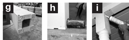
7. All surfaces must be primed, and ends must be sealed with caulk.
