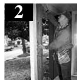
2. Using a jack and post, jack up the beam only enough to remove the existing post and install the new column.
