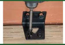
The first deck board needs to be fastened using angle brackets before using the clips. Use Deckmaster Hidden Deck Angle Brackets (HDA), item number DMACP. Fasten the HDA bracket to the bottom of the first deck board, then secure it to the header plate. Using the HDA bracket allows the first deck board to be fastened without screwing down through the top. Use Deckmaster clips once the first board has been installed.
