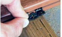
Insert Deckmaster clips into the groove in the deck board at each joist.
