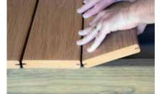
Begin the next board by sliding the board onto the extended leg side of the deck clips. Make sure the new deck board is secured tightly against the deck clips for consistent gapping. Repeat steps 2 and 3.
