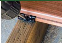
Fasten Deckmaster clips to the joist using the deck screws provided. Slide the screw into the deck clip guide hole and secure at a 45° angle into the joist.
