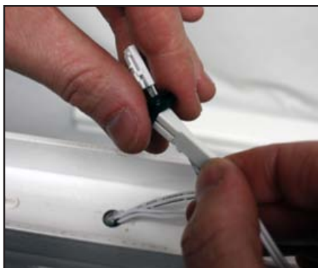
10. Slide grommet over connectors
