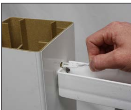
16. On last LED Flush pin on sub-rail run "female" end of LED Flush Pin through hole above bracket into post sleeve
