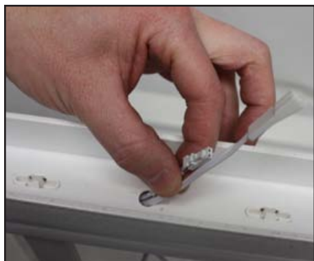
9. Remove grommet and slide wires through sub-rail
