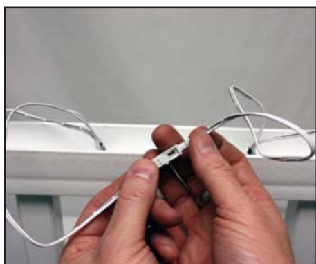
15. Repeat steps 7 through 12, connect "female" end of LED Flush Pin with "male" end of next LED Flush Pin
