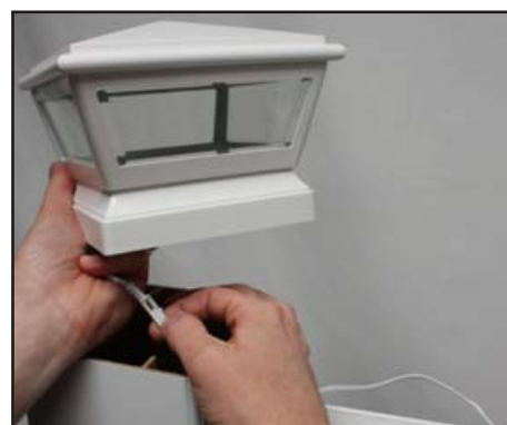
17. Connect "female" end of LED Flush Pin to "male" connector end of Carriage Light LED Post Cap and install Carriage Light LED Post Cap*
