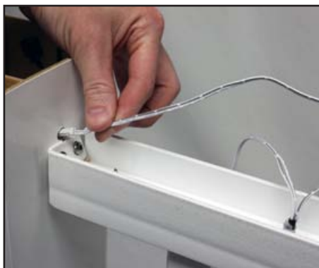
13. Run "male" end of LED Flush Pin wiring through hole above bracket into post sleeve
