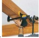
Attach beam side to blocking. The nails
