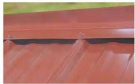
3. Fasten the ridge cap with the Flovent<sup>™</sup> staying in place by the adhesive. Install the ridge cap per the mfg instructions.
