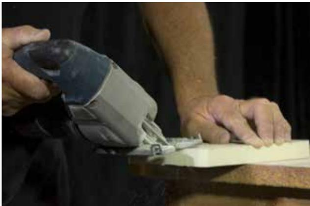
**Step 10** – Now cut the beam top to fit the beam end cap at the same miter angle. Cut at a slight angle to follow the curve of the beam top.
