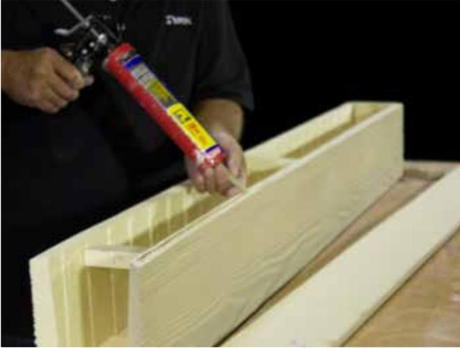
**Step 19** - Now place a thin bead of adhesive (PL Premium®) along the mitered edge of the beam end cap and beam, wipe away any squeeze out of the adhesive.
