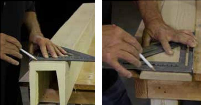
**Step 2** - Square beam using small cut blocks of polyurethane or other material along the length of the beam. This will ensure proper alignment of the beam top.
