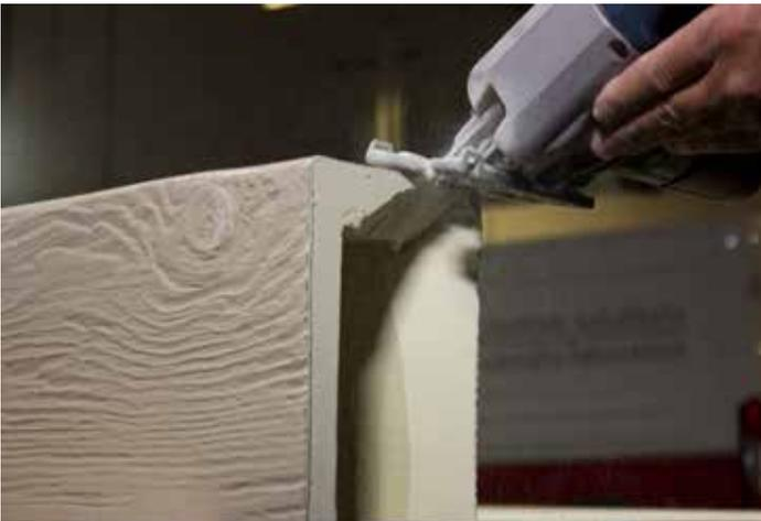
**Step 17** – Again dry fit the beam end cap to the beam and beam top. Determine where you need to sand the beam end cap to achieve a finish fit. Starting with grain side up, use a rasp and/or file to shave the mitered edges on the beam end cap where necessary.
