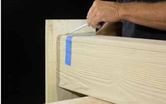
**Step 8** – Using the jigsaw, cut beam end cap along the marked line on the smooth side of the beam end cap.
