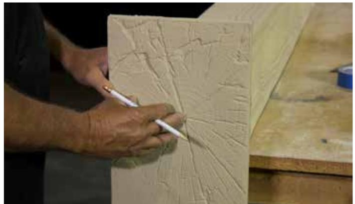
**Step 7** – Holding the smooth side of the beam end cap to the cut beam end and beam top, trace the outline of the beam and beam top onto the end cap.
