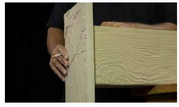
**Step 6** – Holding the smooth side of the beam end cap to the cut beam end, trace the outline of the beam onto the end cap.
