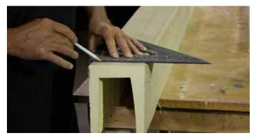
**Step 2** – Using jigsaw with fine tooth blade, cut beam to marked length (cutting all sides of the beam).
