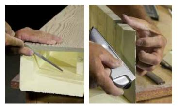
**Step 16** – Again dry fit the beam end cap to the beam. Determine where you need to sand the beam end cap to achieve a finish fit. Starting with grain side up, use a rasp and/or file to shave the mitered edges on the beam end cap where necessary.
