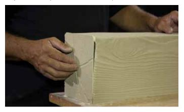
**Step 15** – As you dry fit the beam end cap to the beam, determine where the beam must be filed for the end cap to fit snugly inside the beam. Using a rasp and/or file, shave the interior of the beam miter along the bottom, corners and sides of the beam.
