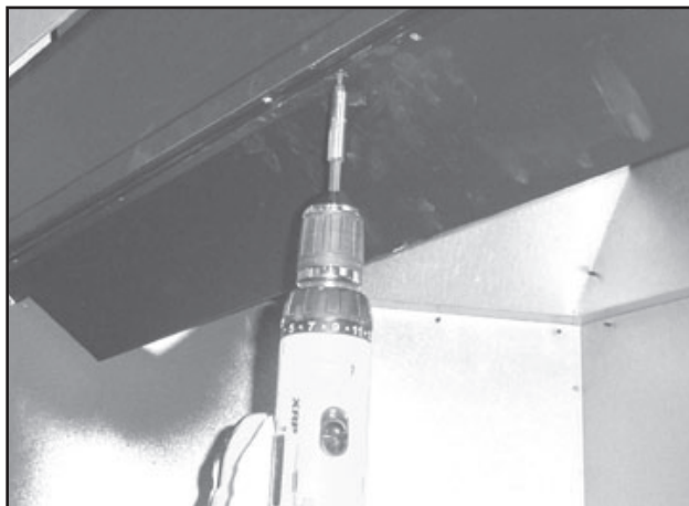
Figure 8.1 Remove Smoke Shield
