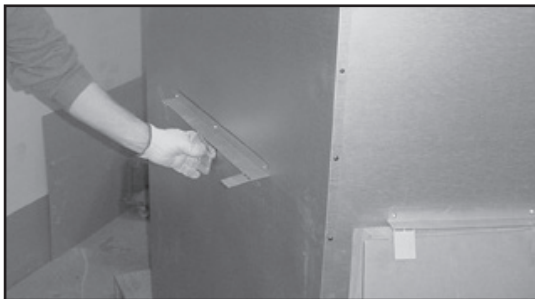
Figure 3.7 Bend Refractory Brackets Back Down
