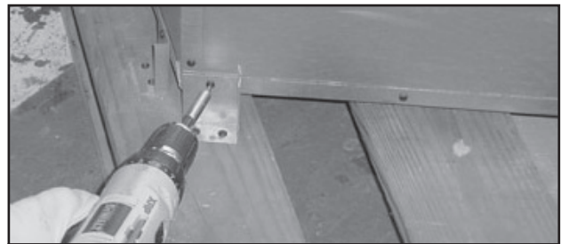
Figure 3.11 Removing Shipping Brackets
