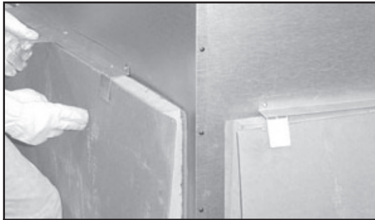
Figure 3.6 Unpack Back Refractory
