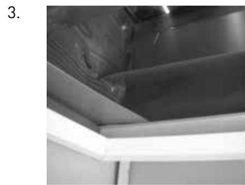
Install Side Cap with a temporary fastener at the gutter end. *(remove protective film from Side Cap before installing)*
