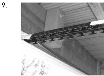
Install remaining carriers with necessary insulators.
