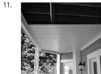
With the carriers installed you can run the panels.
