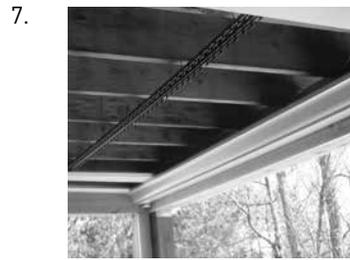
Install gutter to panel height.
