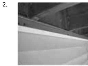
Install G-Channel 1" down from the bottom of the joists. *(remove protective film from G-Channel before installing)*
