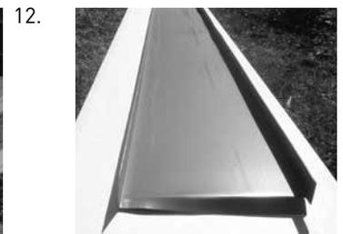
Bend the low end of the panel down into the gutter.
