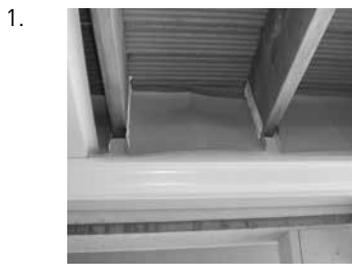
Install pan flashing up inside the joist bays to bring water over the beam into the gutter.
