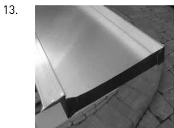
Bend the high side of the panel up to prevent back flow into the G-Channel.
