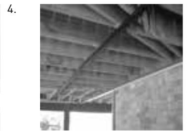
Install the 1st carrier 3 feet from the G-Channel.
