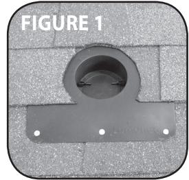
3. At this time the vent hose can be connected to the adapter using a hose clamp or the hose can be connected after installation from the inside of the attic.
