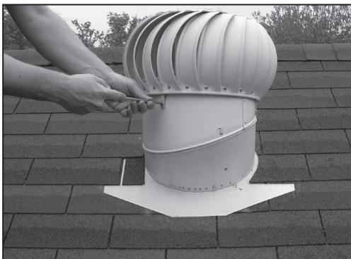
5. Insert a screw through the bracket hole into the new hole in the base and tighten.
