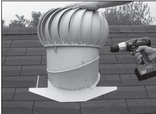
3. Set down gently until brackets on the inside of the turbine head contacts the top edge of the existing base. **CAUTION: DO NOT TRY TO MAKE EXISTING HOLES IN BASE MATCH HOLES IN BRACKETS. THREE NEW HOLES WILL NEED TO BE DRILLED.**
