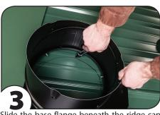
Slide the base flange beneath the ridge cap indicator line on the base flashing. Place 3 ensuring ridge cap completely covers the base flange. Locate base opening between rafters and mark hole to be cut.
