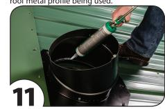
Seal the adjusting seam and the base/elbow connection seam on the inside with roofing cement. Seal locking clamp holes and all exposed screws with roofing cement.
