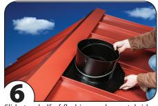
Slide top half of flashing under metal ridge cap while aligning base with cut out. Take care that tape location will ensure good compression and weather tight seal for your roof metal's profile.
