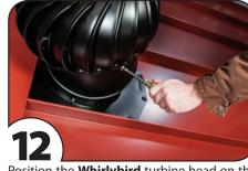
Seal the adjusting seam and the base/elbow Position the Whirlybird turbine head on the connection seam on the inside with roofing base. Line up the predrilled holes in the brackets and elbow and fasten with sheet metal screws.
