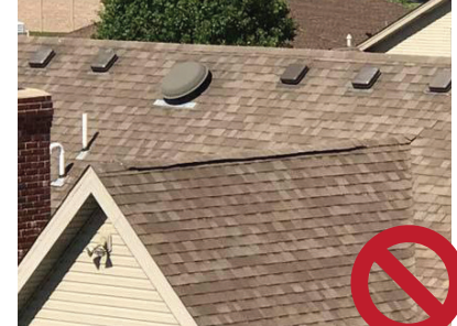
Multiple types of pan-style vents mixed on a roof.
