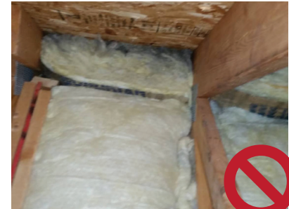
Insulation blockage.
