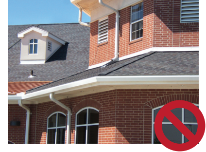
Ridge vent installed on hips.
