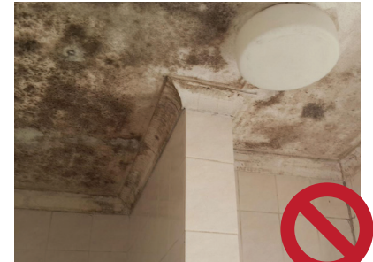
Mold and mildew in a poorly ventilated bathroom.
