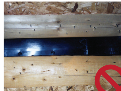
Improper ridge vent opening.
