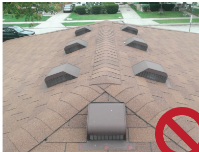
Slant back vents used on multiple sides of a roof.
