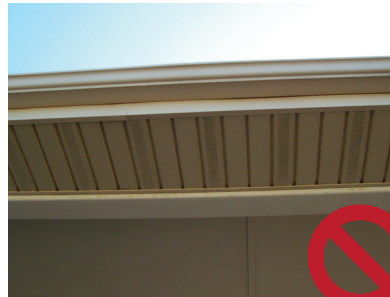
Inadequate soffit panels.
