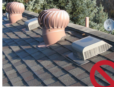
Turbine vents, slant back vents and ridge vent, all on one roof.
