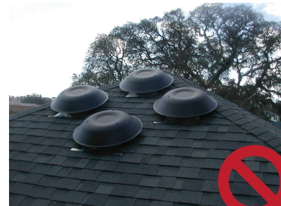
Pan-style vents used at multiple levels on a roof.
