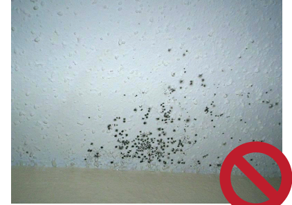
Mold and mildew on an interior drywall ceiling.
