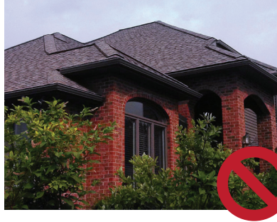
Ridge vent installed on hips.
