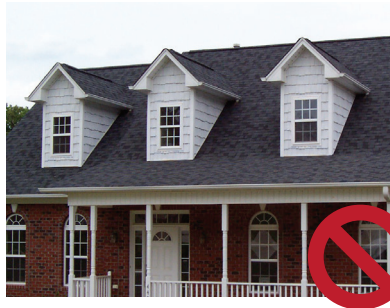
Ridge vent installed on dormers
