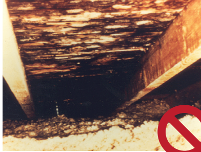
Mold covering wood roof sheathing in an attic.
