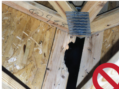
Improper ridge vent opening.
