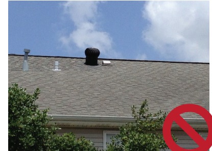
Ridge vent mixed with a turbine vent on a roof.
