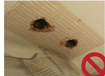
Improper vent openings.
