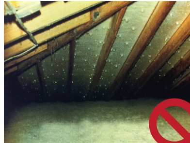
Moisture in the form of frost “raining” on attic insulation as it melts.
