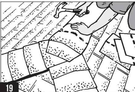
19 Nail all cap shingles in place working from bottom of hips to top of ridge. Finish by capping ridge. Apply a bit of roof sealant to last shingle where needed.
