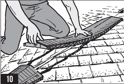
10 Lay HipMaster in position making sure there is good contact with roofing sealant. Ensure that all low points in shingles are filled with sealant. Failure to properly seal could lead to water intrusion.
