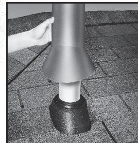
2. Place CapMaster over pipe and rotate to proper angle. Friction clips hold it in place.
