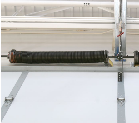
Heavy-duty torsion spring system
