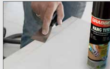
4. Apply Grabber adhesive and press down paper using finishing tool
