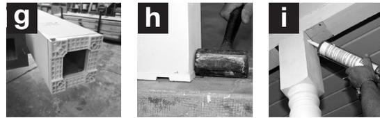
7. All surfaces must be primed, and ends must be sealed with caulk.
