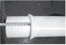
Slide the mid-trim ring onto the post, as shown. 8" and 10" tapered posts have an offset on which the ring rests. The location of the rings for straight posts should be predetermined (typically, 8" from the top on the 8" post) and
