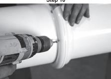
With the rings properly positioned on the 8" straight post, drive #8 x 2" self-drilling screws into the post through the holes in the top of the ring, as shown. Slide the top and bottom trim over the post, followed by the top and bottom mounting brackets.
