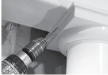
Top trim is now fixed to the carrying beam as shown using #8 x 2" self-drilling screws.
