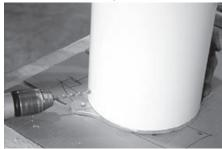
In areas where uplift from high winds is considered a problem, pre-drill ½" holes through the column and bracket ears at the position of the bracket mounting tabs into the post approximately 1" from the bottom and 1" from the top.
