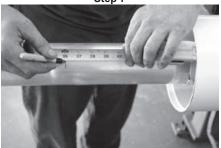
Before pre-assembling column, you must determine the placement of the spacers. Measure from the bottom of the aluminum insert (34" for 36" high railing and 40" for 42" high railing). This will be the placement of the bottom of the aluminum insert spacer.
