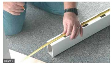
5. Cut rail to size and then place both bottom rail multi-angle connector brackets onto the rail. Slide the rail into place and temporarily connect the multi-angle connectors and pivot brackets together (Fig. 7). Make sure the spindle holes are evenly spaced between the mounting surfaces. Once properly aligned mark the multi-angle connector bracket location on both ends and remove the rail. (Note: Cut evenly from both ends and the top rail should be cut to the same length as the bottom rail).
