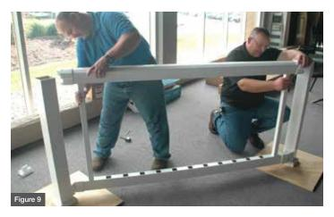
9. Line the pivot bracket up with the multi-angle connector and center on the post and mark the placement (Fig. 10 & 11).
