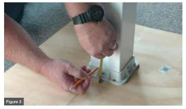
2. Place the pivot bracket on the mark and center on the post. Mark the openings in the bracket on the post, predrill the post on marks (Fig. 4).
