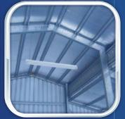
R+HEATSHIELD radiant barrier is made from a woven polyethylene material covered by a metalized film, which blocks up to 94% radiant heat. R+HEATSHIELD also meets the requirements for Sensitive Compartmented Facilities (SCIF) applications, providing an effective attenuation barrier against a wide range of RF frequencies.
