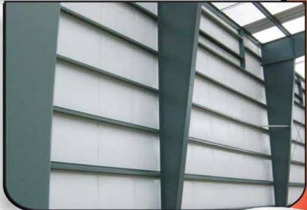
**rFOIL286**<sup>™</sup> Reflective Insulation is a single layer of ¼" high-strength polyethylene bubble, bonded to and sandwiched between a layer of metalized aluminum film, with an interior facing of UV-Resistant polyethylene.
