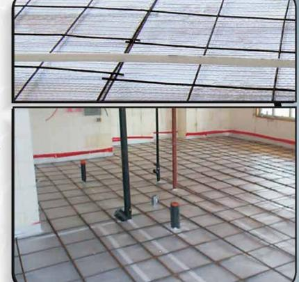
**rFOIL**<sup>™</sup> **Concrete Underpad** is an outstanding reflective insulation and puncture-resistant vapor barrier. It is composed of a double layer of high-strength polyethylene bubbles (up to 60 psi), sandwiched between one layer of metalized aluminum, and a layer of white polyethylene.
