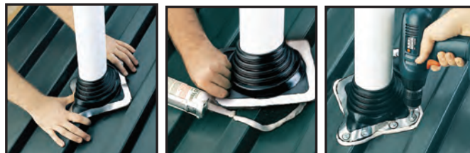
3. Form to roof profile 4. Apply sealant 5. Fasten to complete
