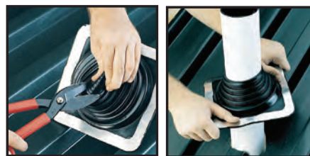
1. Choose pipe opening and trim 2. Slide over pipe
