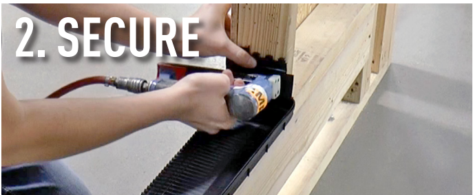
2. SECURE Place the sill pan in the rough opening and secure it into place utilizing screws or staples.
