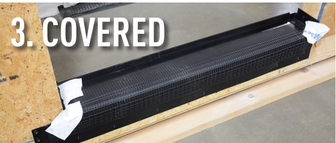
3. COVERED Fully seal corners with provided flashing tape and rest assured – you're covered.
