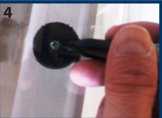
4. Place your cover over the well. Use a marker to mark the location of the Dual-Lock™ disc. You will use this mark to attach the corresponding Dual-Lock™ pad to the underside of your cover. Clean the area under the cover before you adhere the Dual-Lock™ Pads
